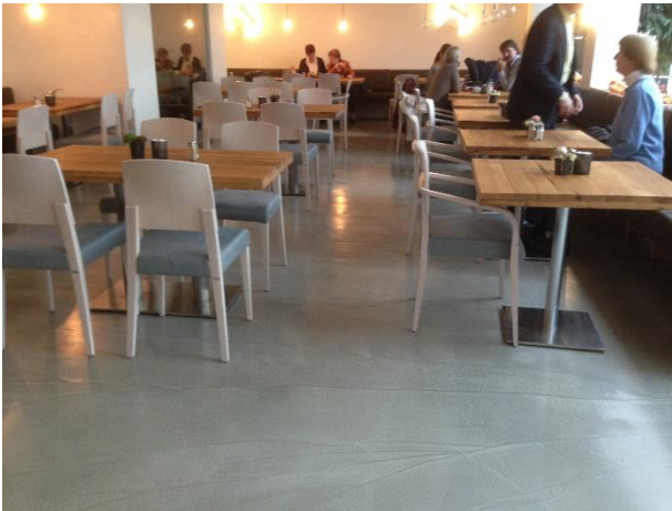
Picture 1, Restaurant of a hotel, renovation during operation
