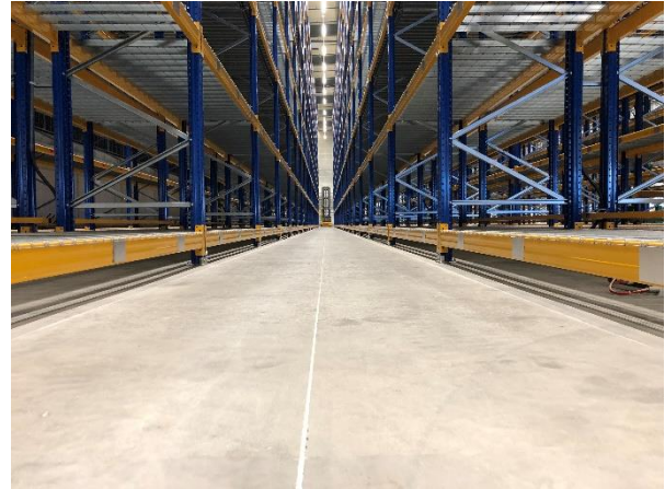
Figure 11, High-bay warehouse for water-polluting substances, production area for water-polluting substances
