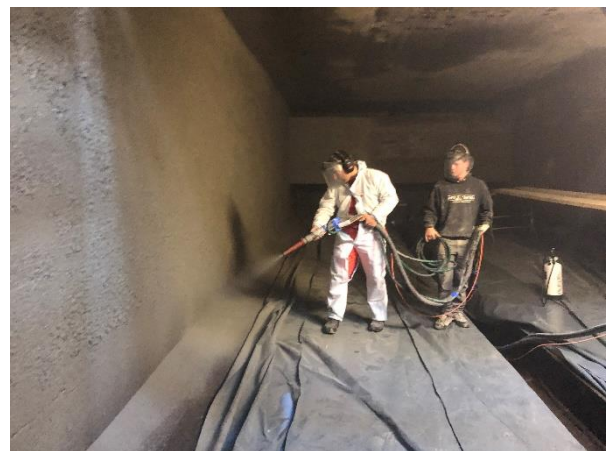
Figure 12, reprofiled concrete in industrial sewage treatment plant according to WHG
