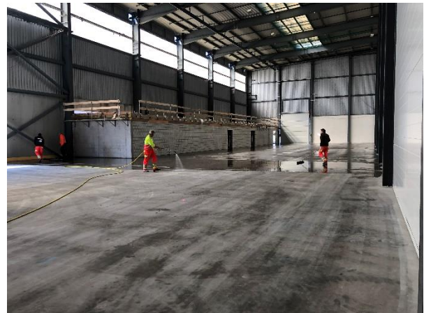
Figure 7, Industrial concrete floor for intensive forklift access, spray application after cleaning
