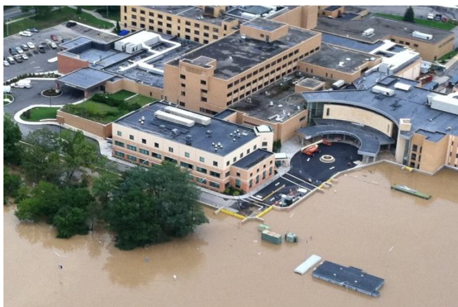
Floodwall protected Our Lady of Lourdes Hospital in Binghamton, Broome County, New York.
